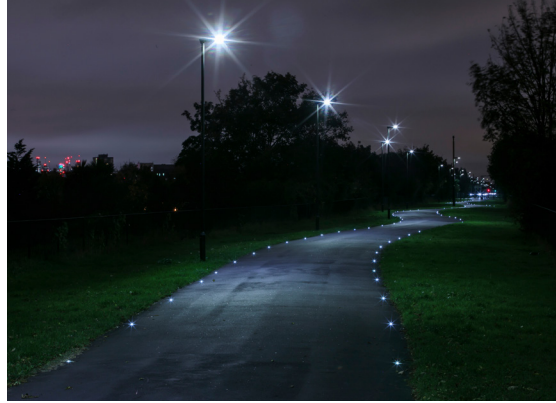
Newham Greenway - edge installation
